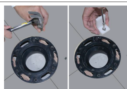
6. Insert the plastic sleeves, attach the seven-type mounting brackets and install the floor screws.
