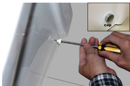
10. Tighten the toilet bowl mounting screws and then put on the caps.
